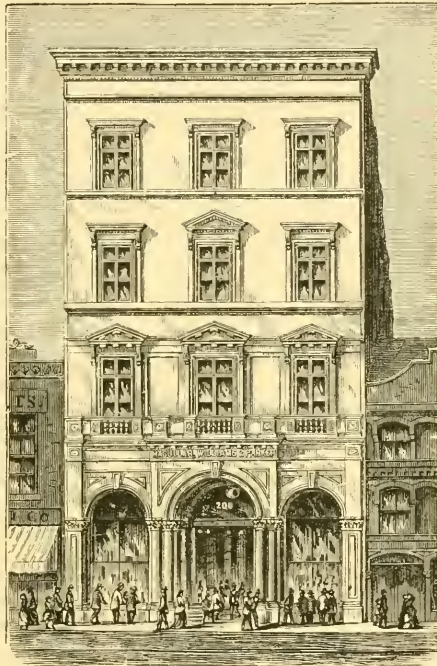
MACULLAR, WILLIAMS & PARKER'S BUILDING IN 1872
